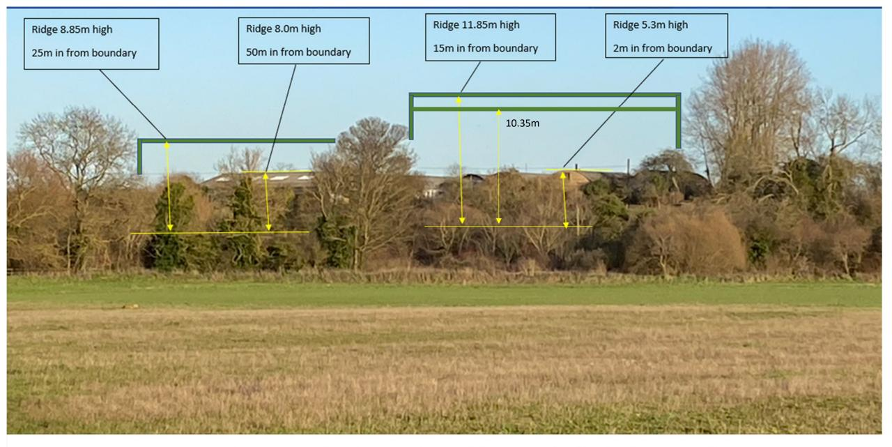
Proposed profile above existing buildings to scale allowing for perspective
